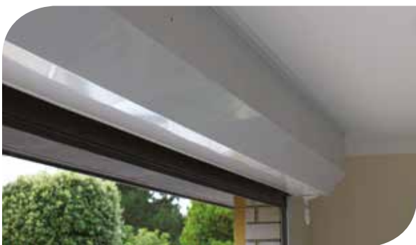
Internal view showing canopy (box)
