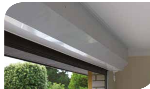
Internal view showing canopy (box)
